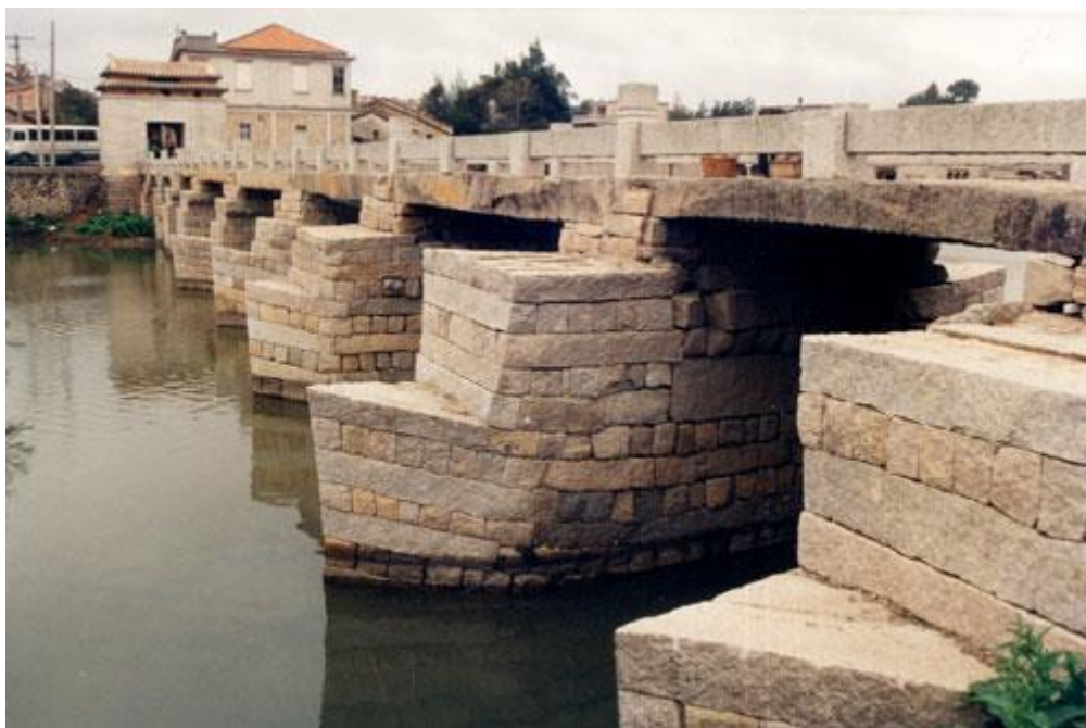
泉州安平桥的桥墩分水尖
